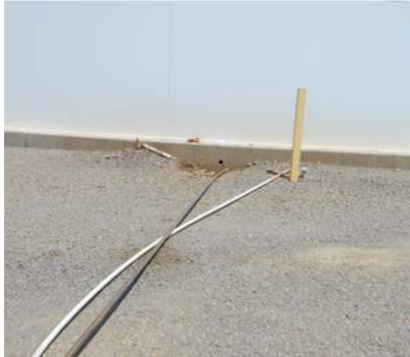
Core Drilling to install new reference electrode.
