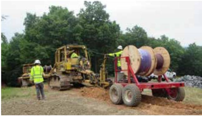
**Figure 3. Cable plow installation of linear anode to the side of the pipeline along the ROW.**
