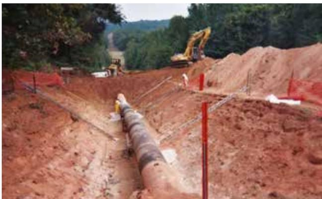
Figure 2. Recoating operation along the open right-of-way (ROW).
